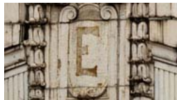
Photos: Everyman Theatre renovation
